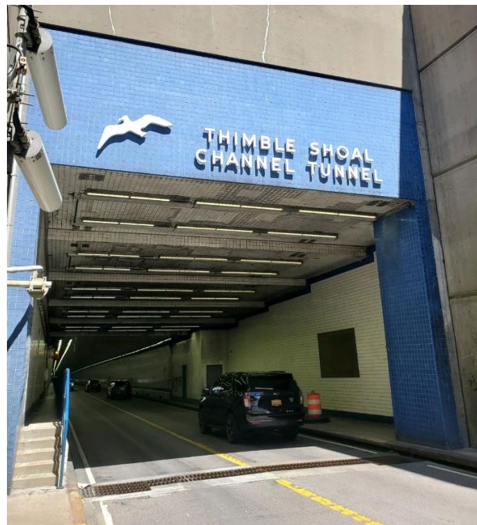
Figure 6– Thimble Shoal Tunnel Portal
