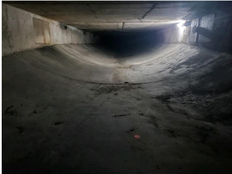
Figure 10 - Typical Lower Air Plenum
