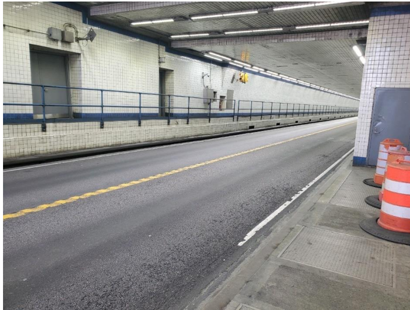
Figure 8 - Typical Tunnel Roadway with Catwalk
