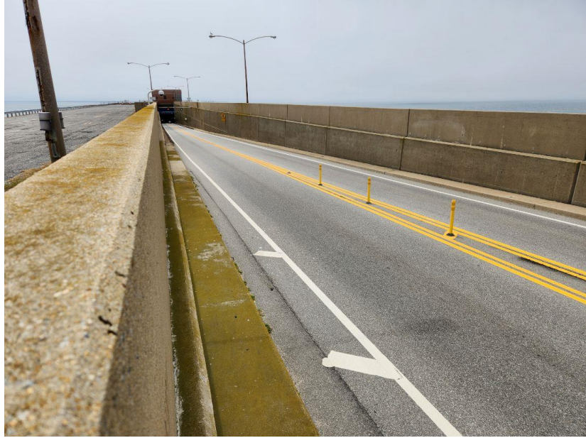
Figure 9 - Typical Open Cut, Leading to Tunnel Portal
