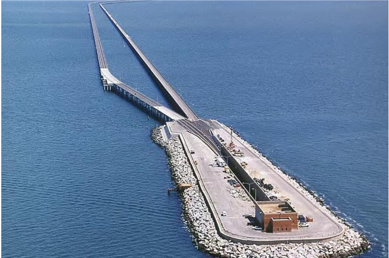
Figure 2 – Portal Island No. 4 and Trestle CSB (l) and Trestle CNB (r)
