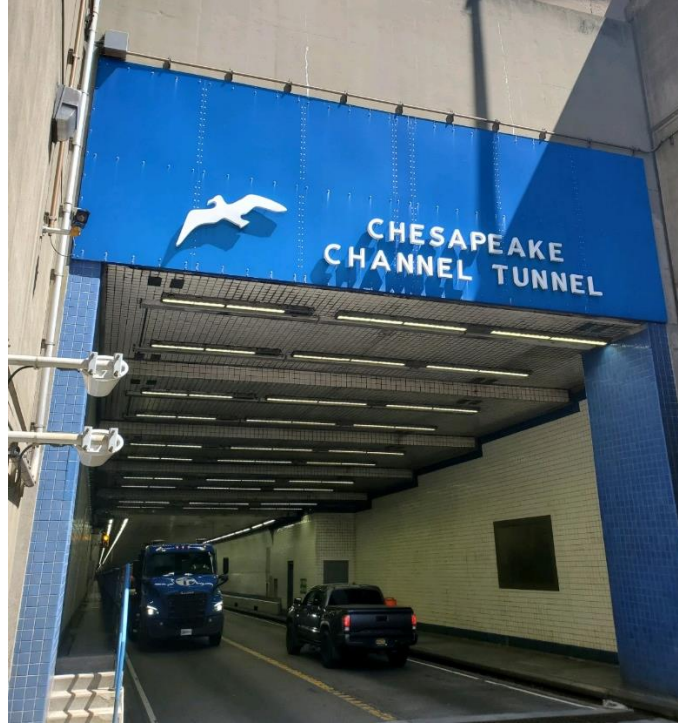
Figure 7 - Chesapeake Tunnel Southern Portal
