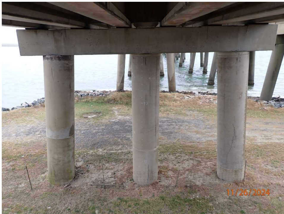
Photo 66: FNB6 Substructure in good condition.
