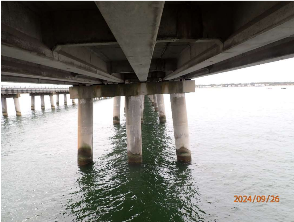
Photo 12: ASB67 typical substructure elevation. Substructure elements typically in good condition.
