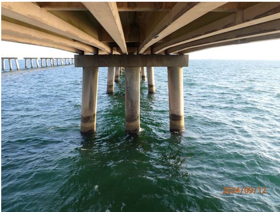
Photo 16: BNB178 – superstructure and substructure in good condition.
