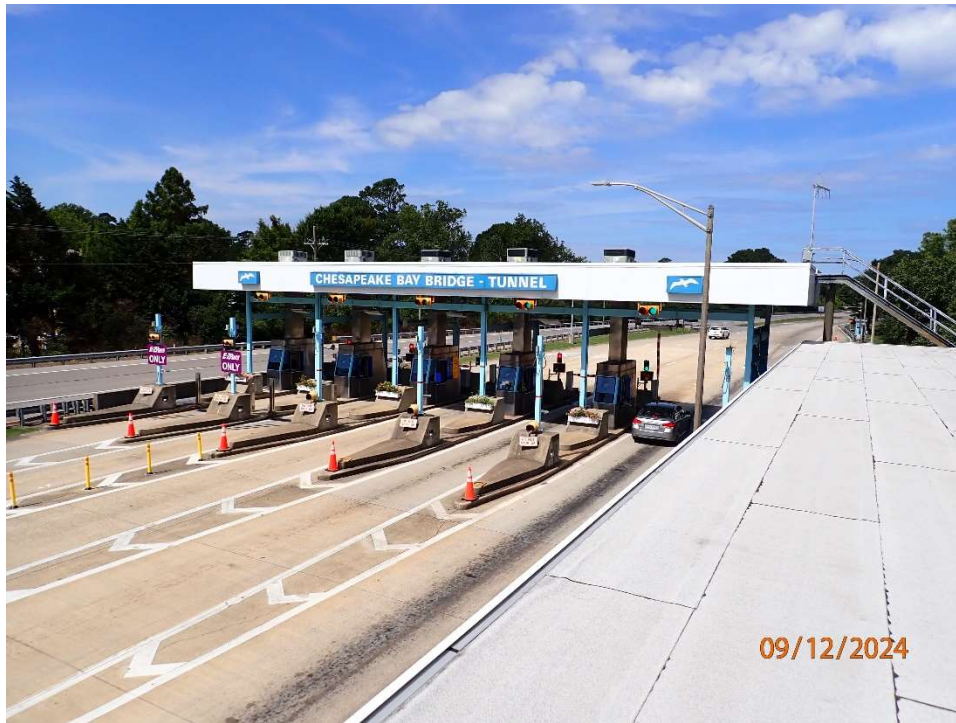
Photo 120: South Toll Plaza; Toll Booth Plaza in good condition.
