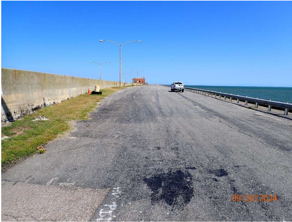
Photo 106: Portal Island 3; Surface; Typical pavement condition on east side of island.
