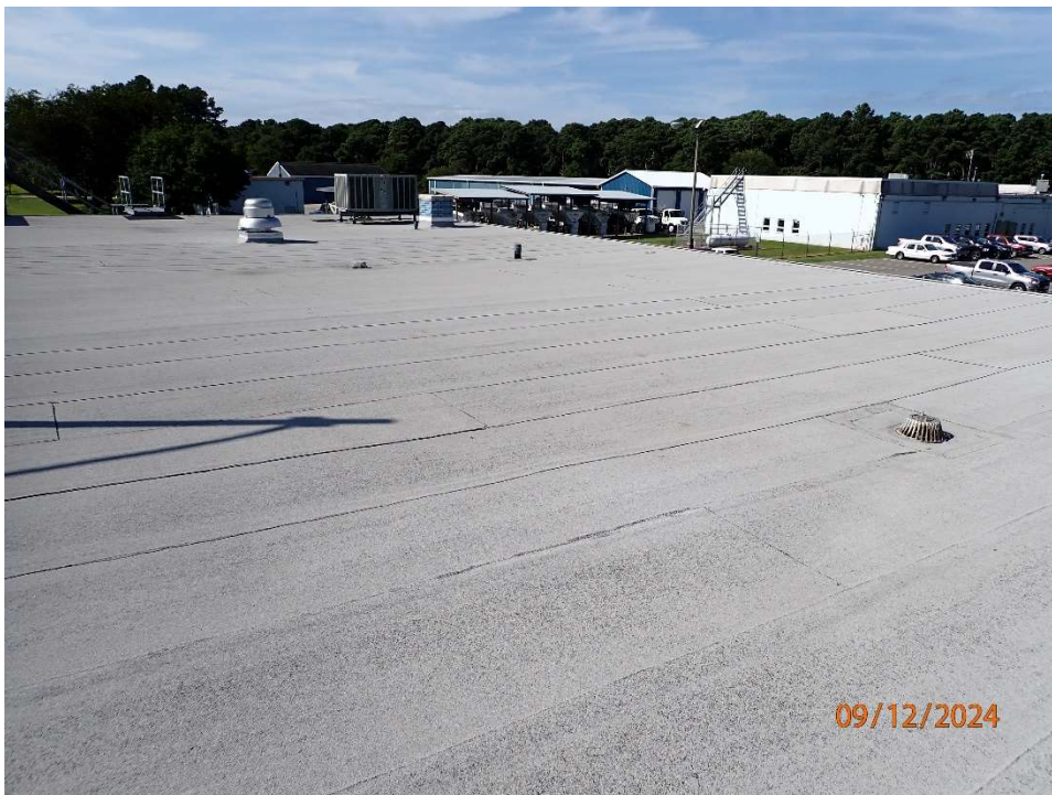
Photo 125: North Toll Plaza, Toll Office Building roof in good condition.
