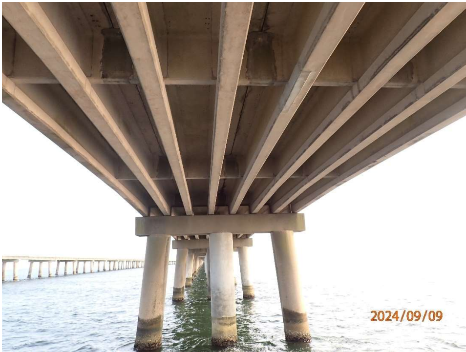
Photo 4: ANB177 – Typical Superstructure & Substructure in good condition.
