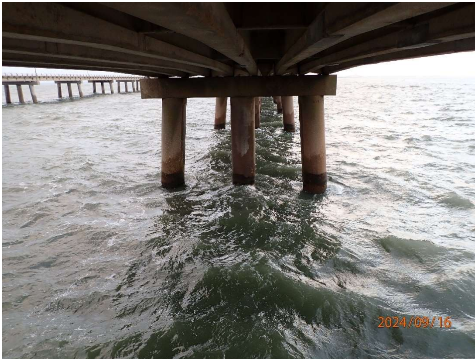
Photo 27: CNB198 Superstructure & Substructure in good condition.
