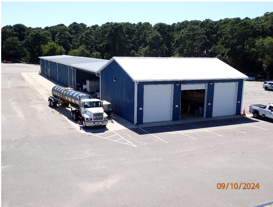
Photo 137: North Toll Plaza, Equipment Storage Building in very good condition. Minor damage noted to Bay 2 trim on north storage structure.
