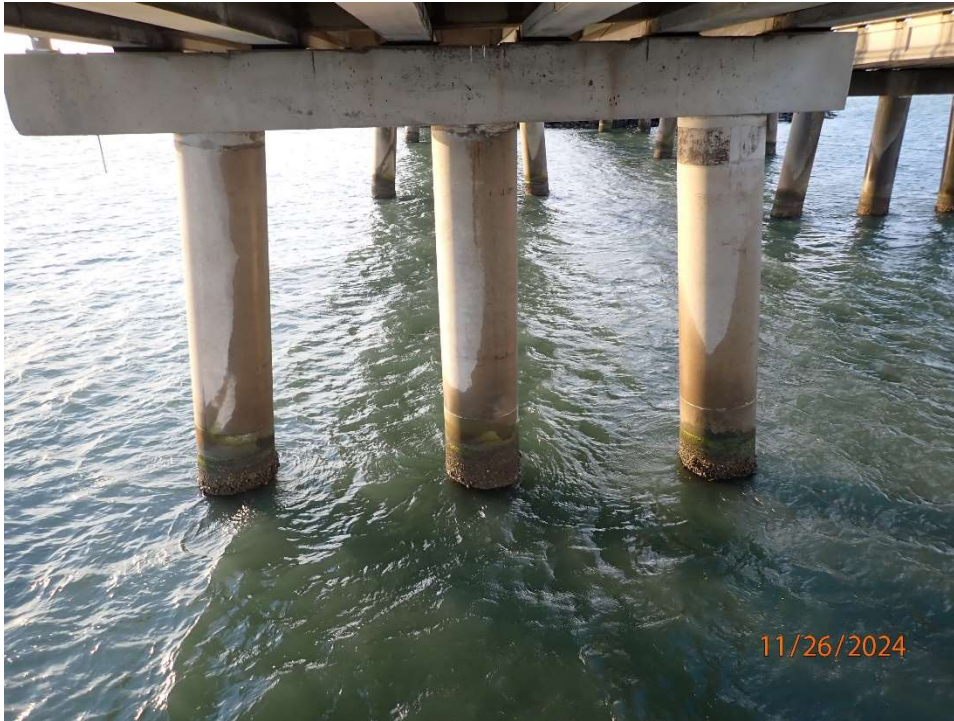
Photo 61: ENB4 Substructure in good condition.
