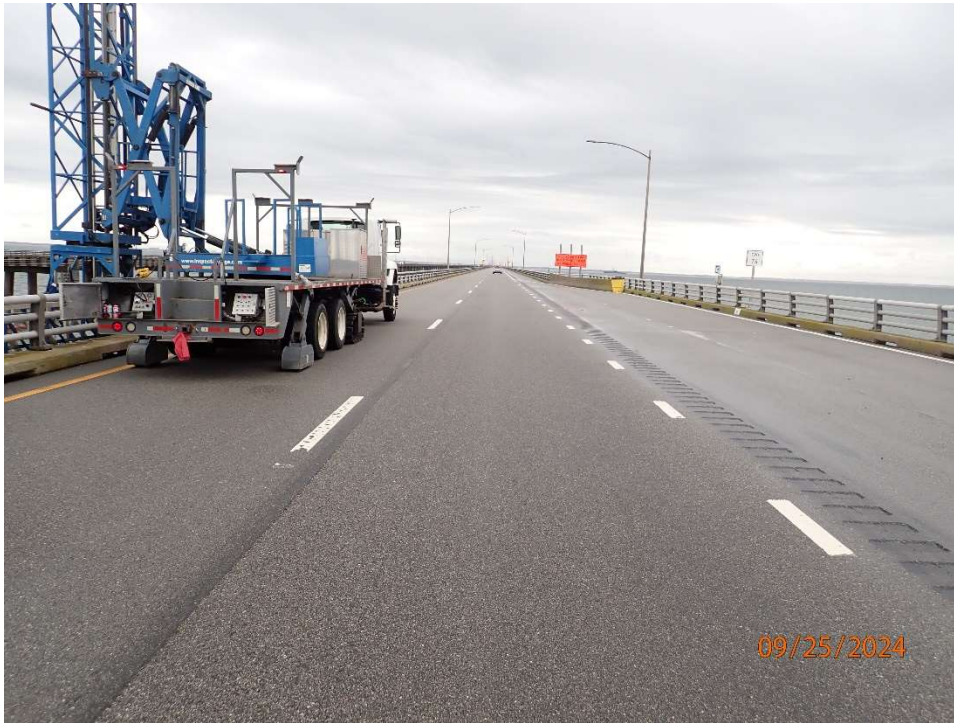
Photo 21: BSB100 Deck Wearing Surface in good condition and inspection equipment mobilized.
