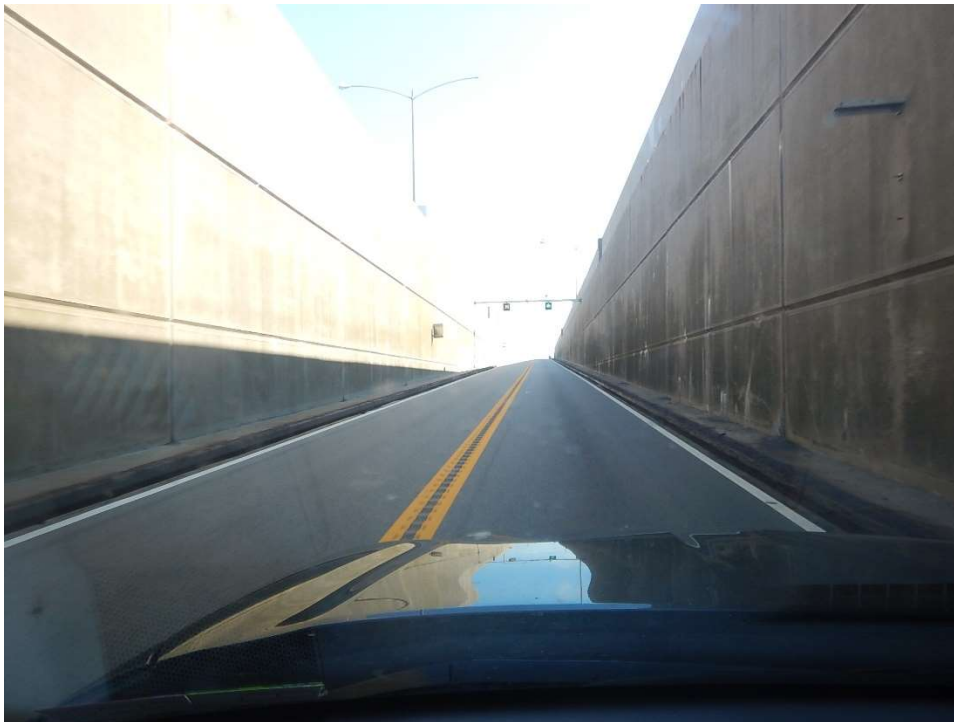
Photo 78 – Island 4 Open Approach Roadway (Looking North)
