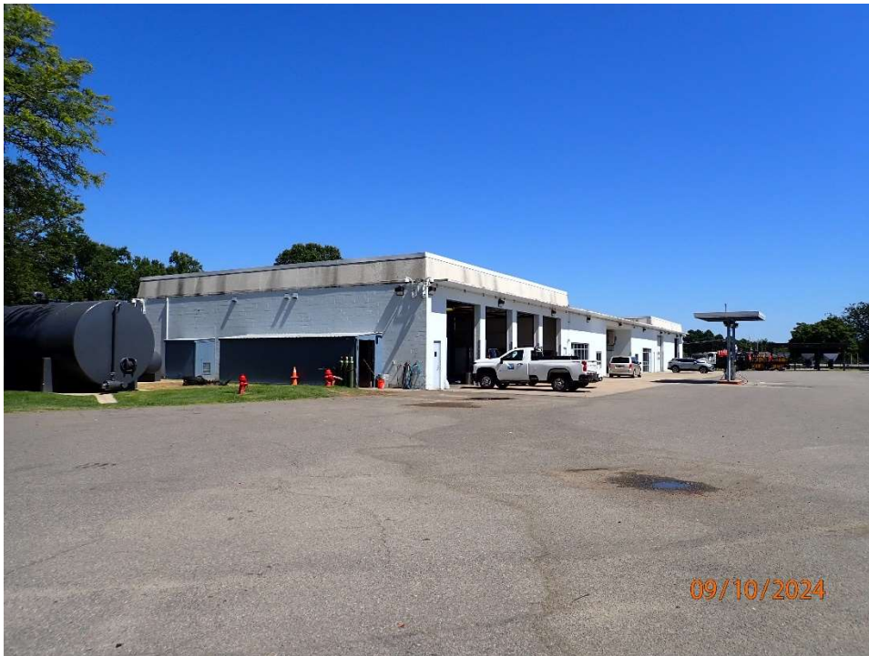
Photo 133: North Toll Plaza, Maintenance Building in overall in good condition.
