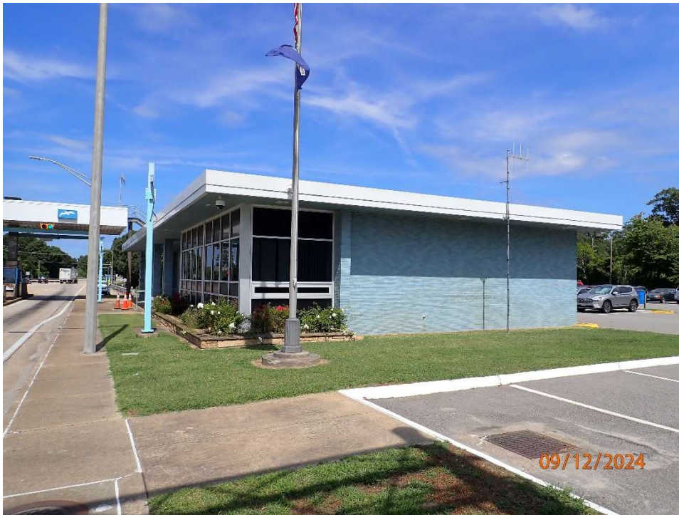
Photo 118: South Toll Plaza; Toll Office Building
