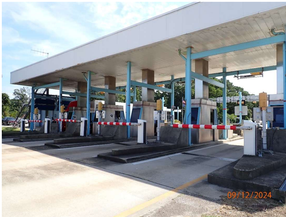
Photo 121: South Toll Plaza; Toll Booth Plaza in good condition.
