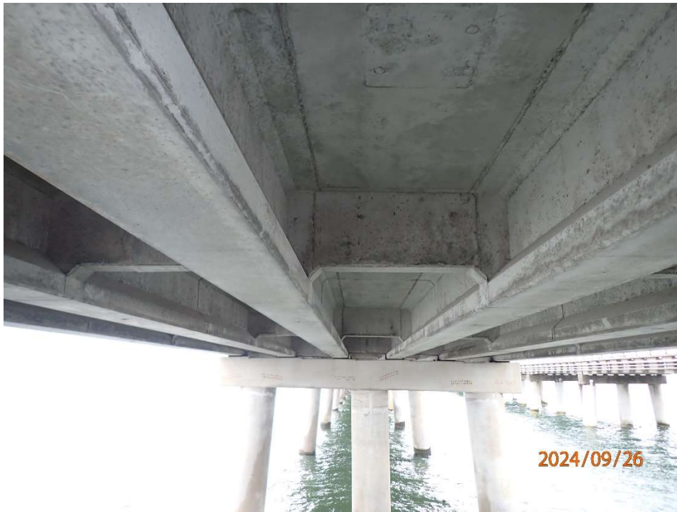
Photo 23: BSB96 Substructure in good condition.
