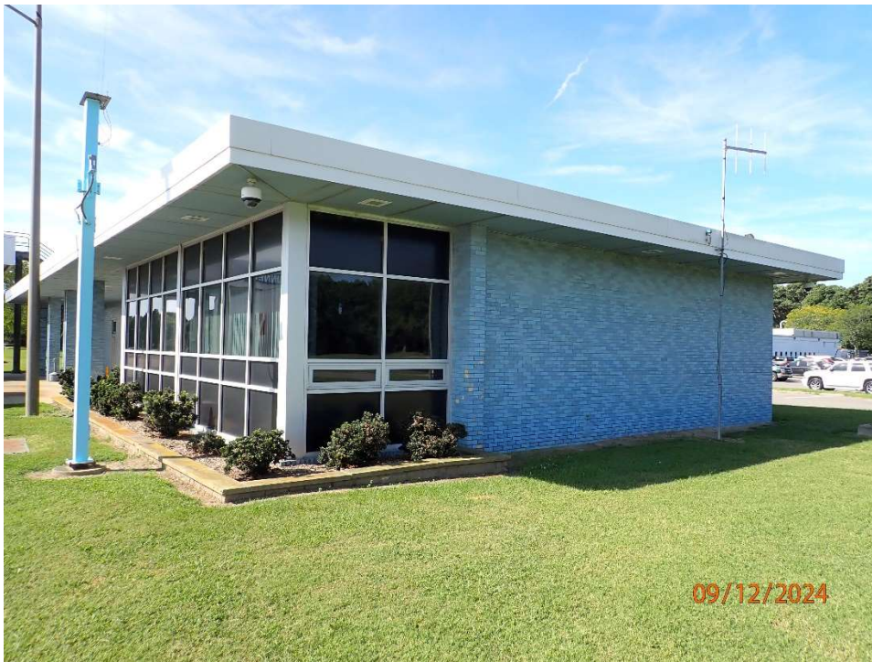
Photo 124: North Toll Plaza, Toll Office Building
