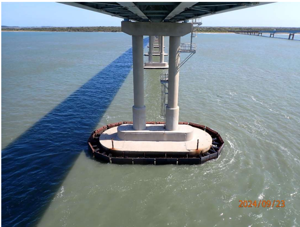
Photo 41: Fender System – Typical Condition of Pier Footing and Fender System.
