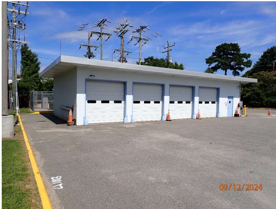
Photo 122: South Toll Plaza; Garage in good condition.
