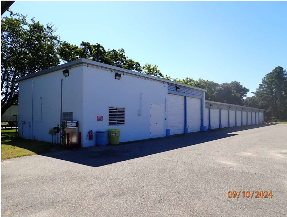
Photo 134: North Toll Plaza, Garage & Generator Building in overall in good condition.
