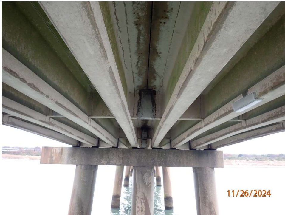
Photo 49: Superstructure and Substructure – Typical condition of Superstructure in Span 1 looking North.
