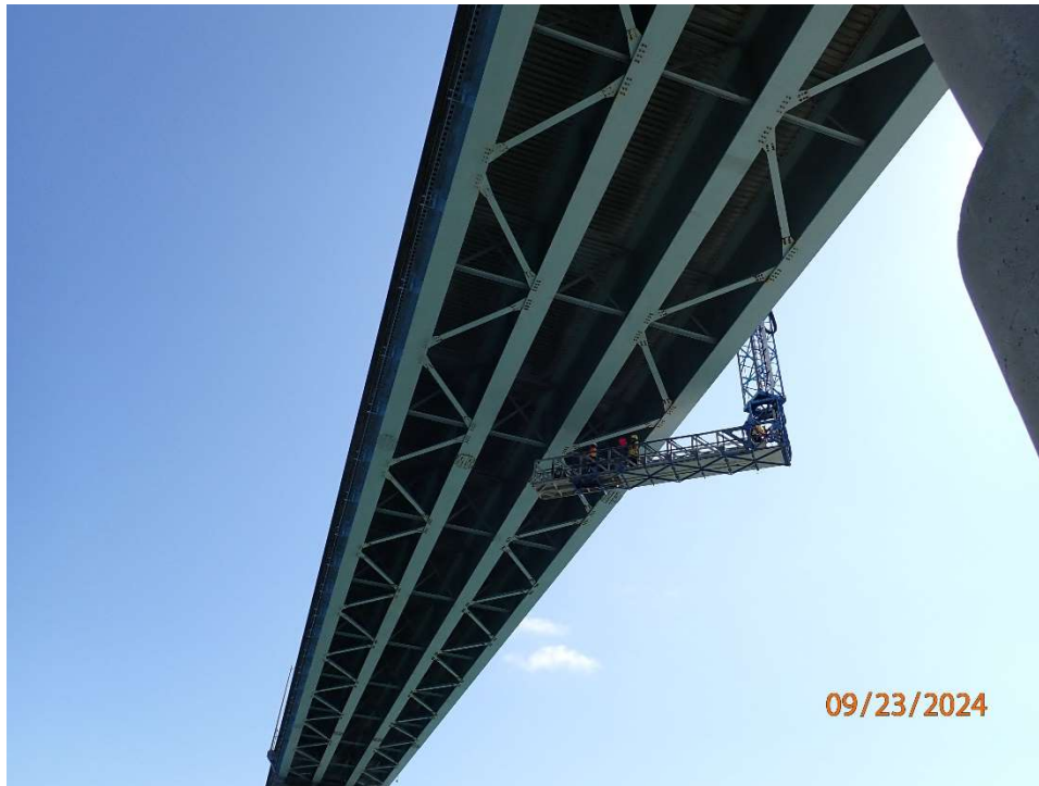
Photo 38: Superstructure – General Condition of Steel Superstructure
