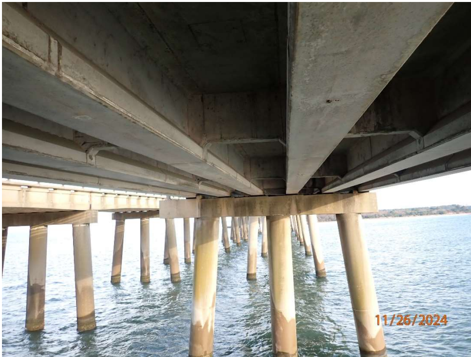
Photo 62: ENB5 Superstructure in good condition.
