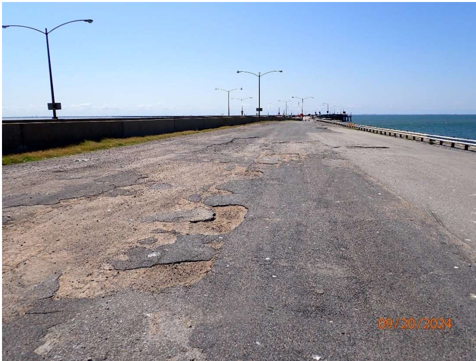
Photo 107: Portal Island 3; Surface; Typical pavement condition on west side of island.
