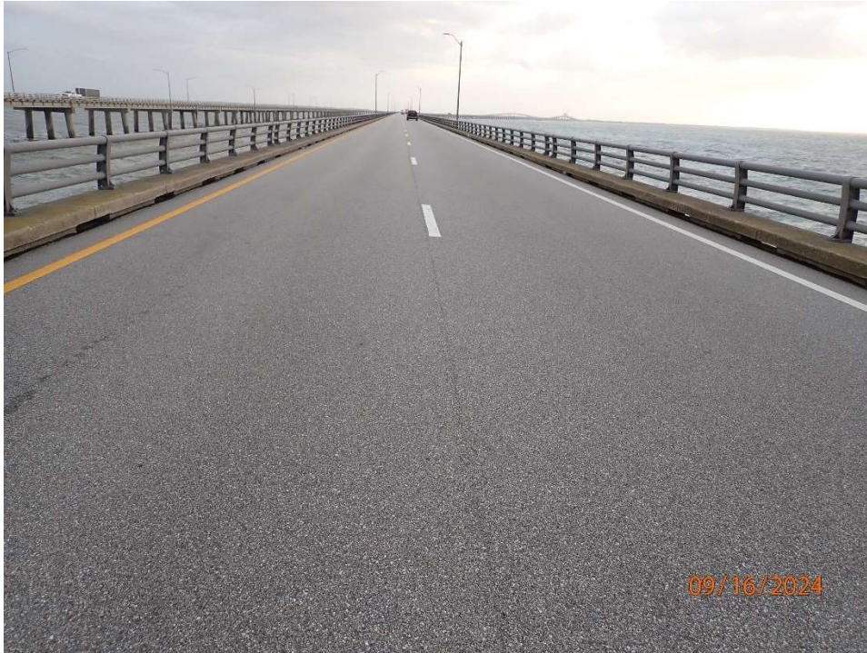
Photo 24: CNB199 Asphalt Wearing Surface – Typical Good Condition of Wearing Surface.
