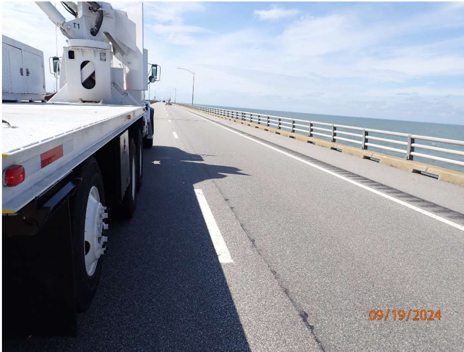
Photo 32: CSB97 Top of deck in good condition.
