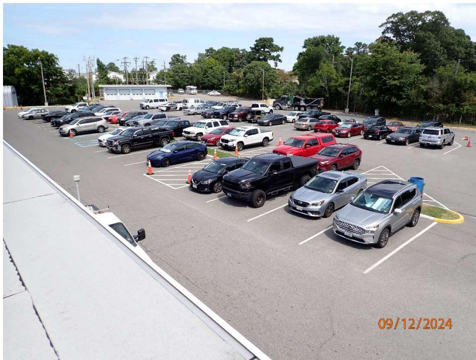
Photo 123: South Toll Plaza Parking Lot; Pavement has isolated alligator cracking up to 1/8" wide; however, overall, in good condition.
