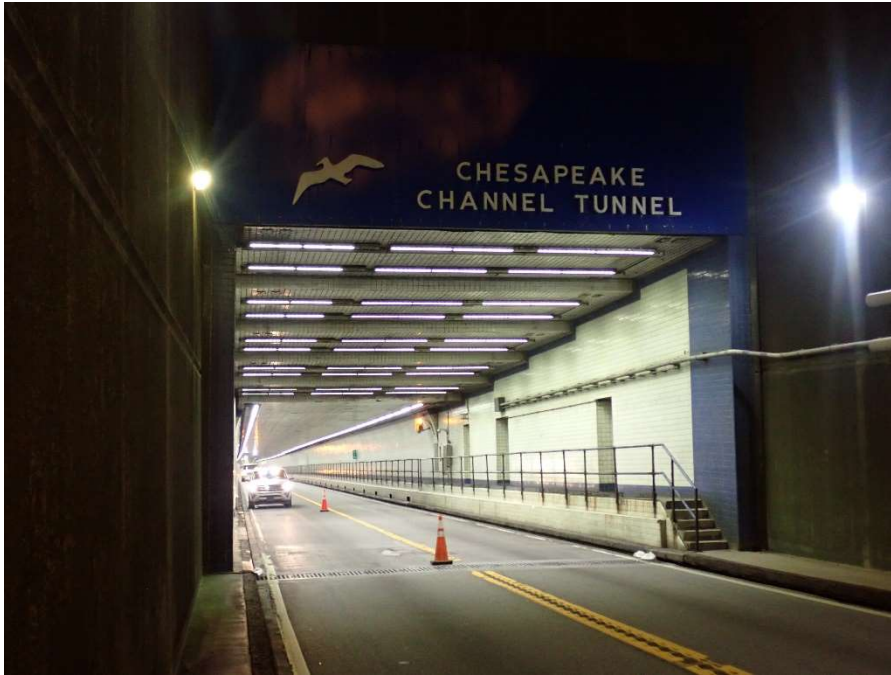
Photo 81: Tunnel Portal – General View of Island 4 Portal (Looking South)
