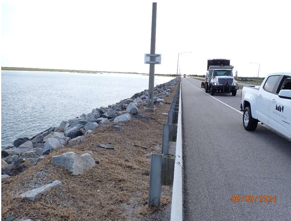
Photo 101: FIB Causeway headed north (looking south); Typical shoreline stabilization.
