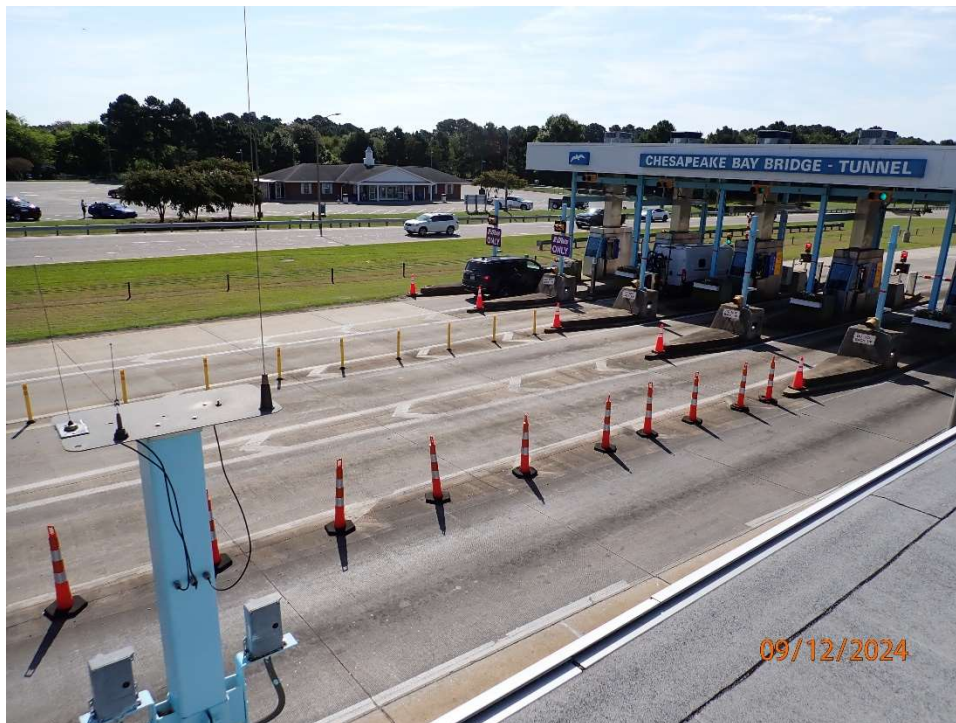
Photo 127: North Toll Plaza, Toll Booth and Canopy with roadway approach in good condition.
