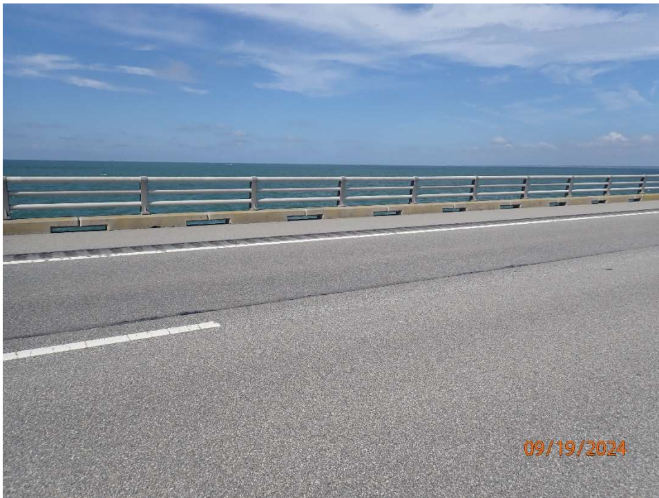
Photo 33: CSB90 Metal Bridge Railing— Typical Good Condition of Bridge Railing.
