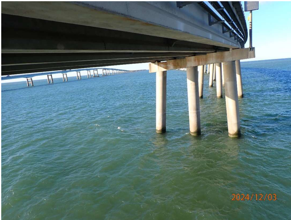
Photo 57 – DSB9 Bent in good condition (typical)
