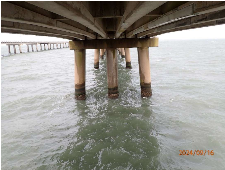
Photo 29: CNB213 Superstructure & Substructure in good condition.
