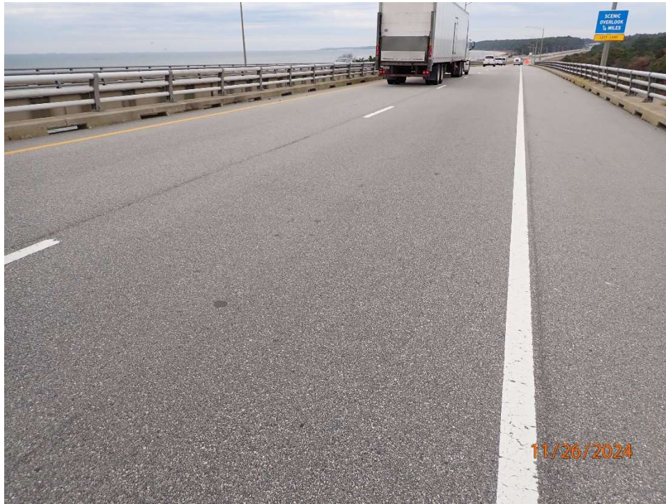
Photo 59: FNB2 - Wearing surface in good condition.
