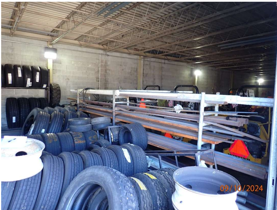
Photo 135: North Toll Plaza, Garage & Generator Building with interior in good condition with signs of minor leakage on backwall.
