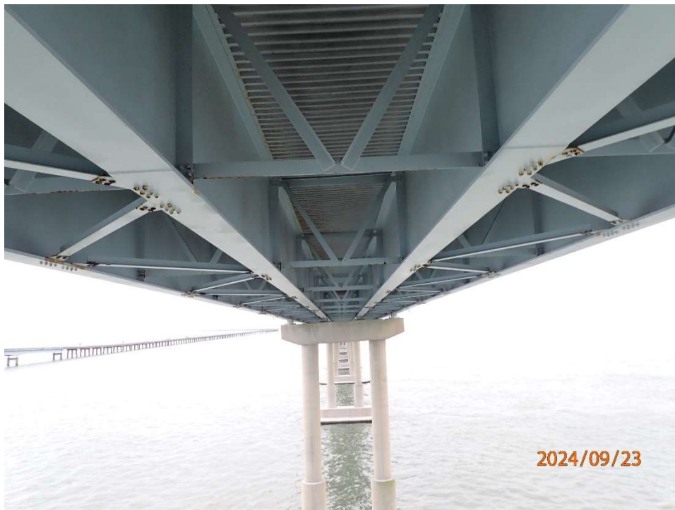
Photo 39: Superstructure – General Condition of Steel Superstructure in fair condition.
