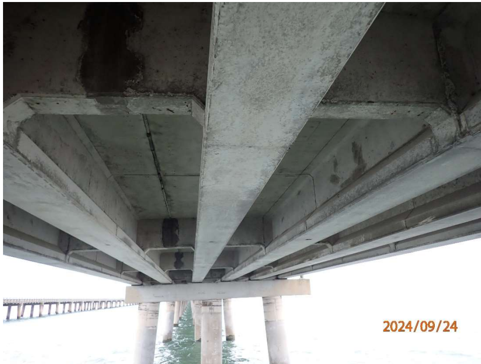
Photo 34: CSB91 Superstructure and Substructure in good condition.
