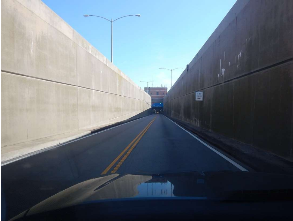
Photo 77 – Island 3 Open Approach Roadway (Looking North)
