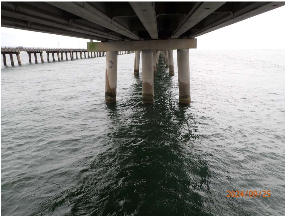
Photo 22: Superstructure in good condition.
