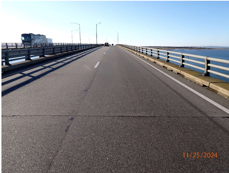
Photo 68: FSB4 Wearing surface in good condition.
