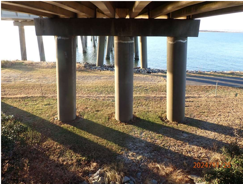
Photo 71: FSB4 Superstructure and substructure in good condition.
