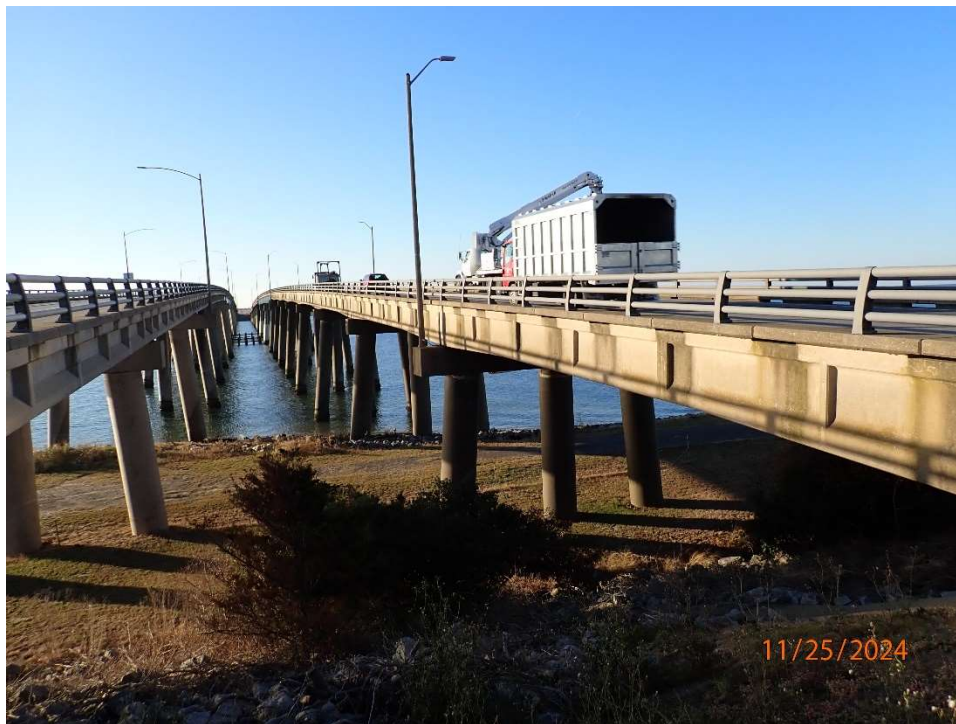
Photo 60: Elevation view of FIBNB and FIBSB.
