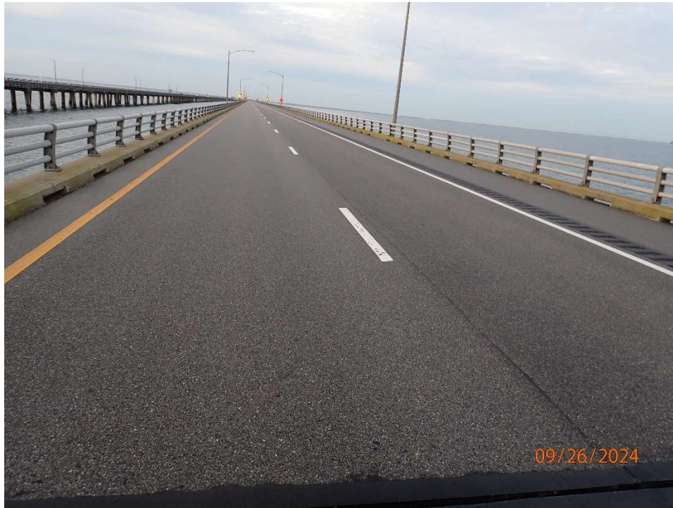
Photo 10: ASB50 Asphalt Wearing Surface – Typical Good Condition of Wearing Surface
