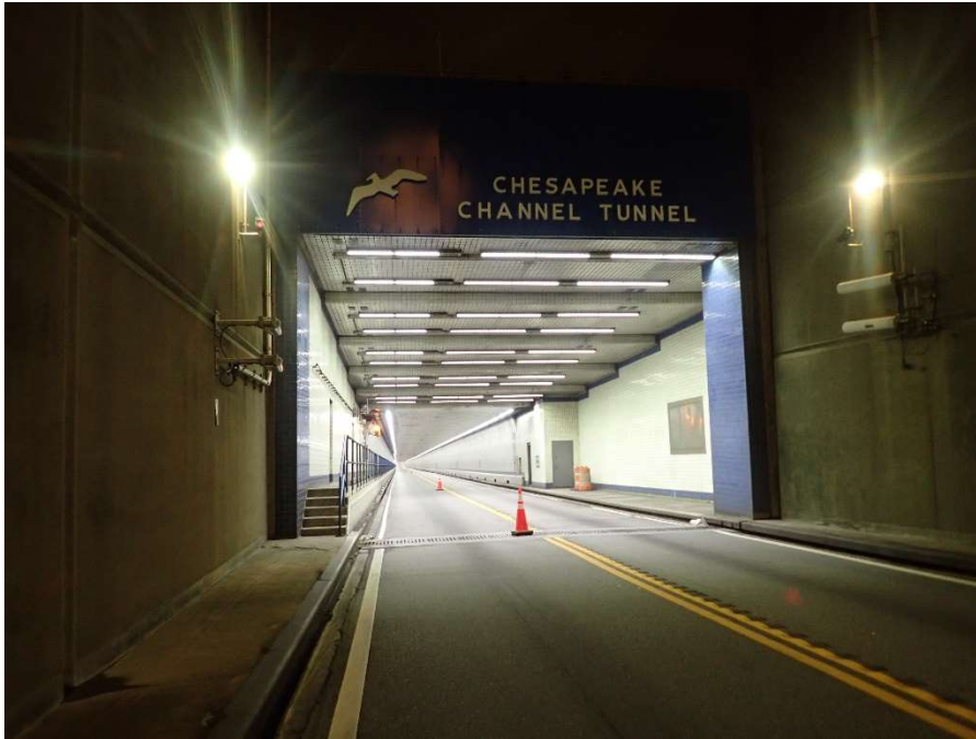
Photo 79: Tunnel Portal – General View of Island 3 Portal (Looking North)
