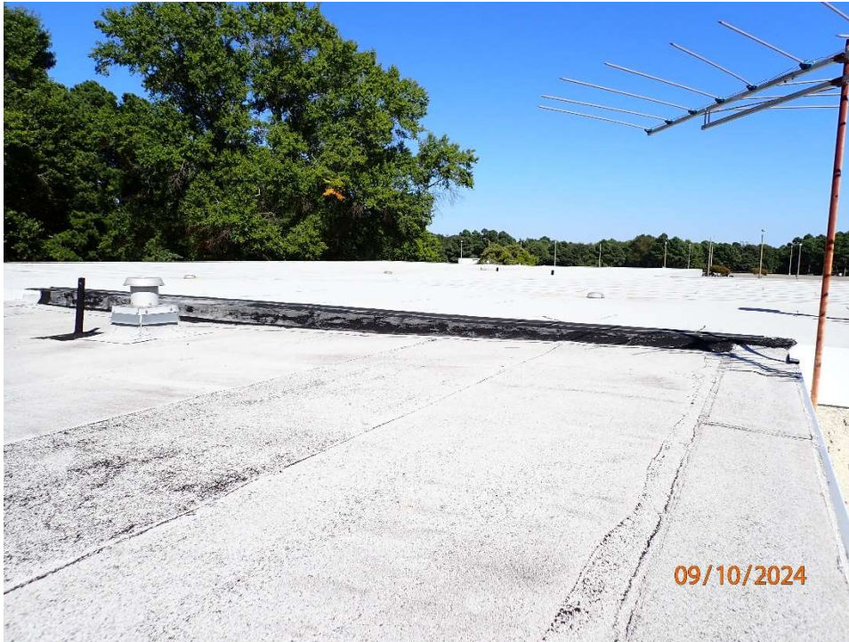
Photo 132: North Toll Plaza, Administration Building roof in good condition.
