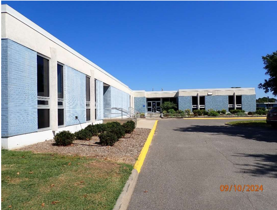
Photo 130: North Toll Plaza, Administration Building in good condition.
