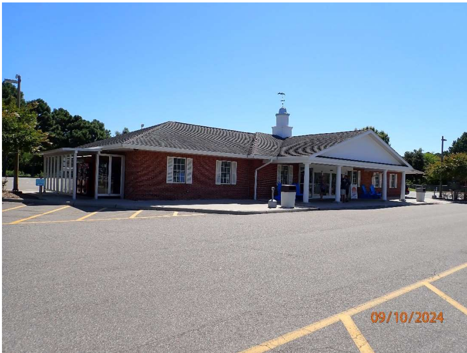
Photo 139: North Toll Plaza, Rest Room Facility in good condition with alligator cracking noted throughout the parking lot.
