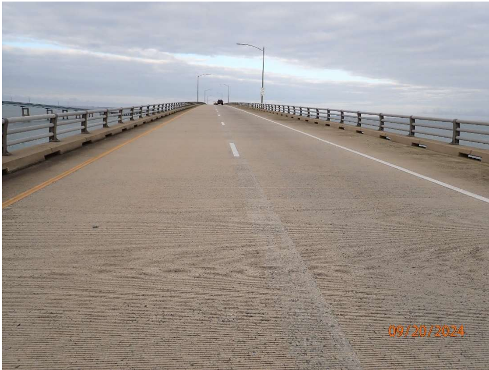
Photo 36: NCB-SB Deck and Wearing Surface – General Good Condition (Looking South)
