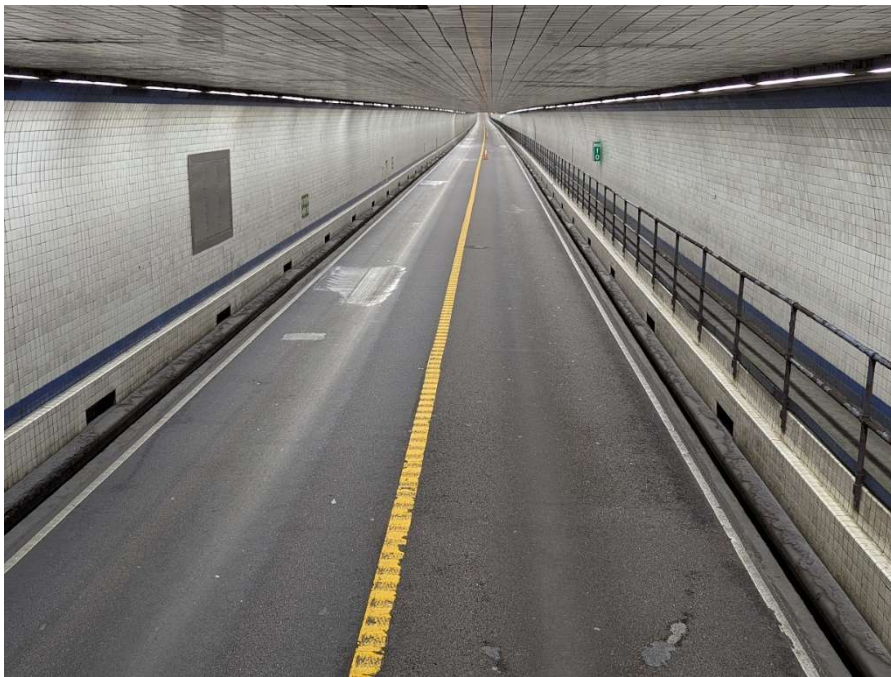
Photo 82: Tunnel Roadway – General View along Tunnel Roadway (Looking South)
