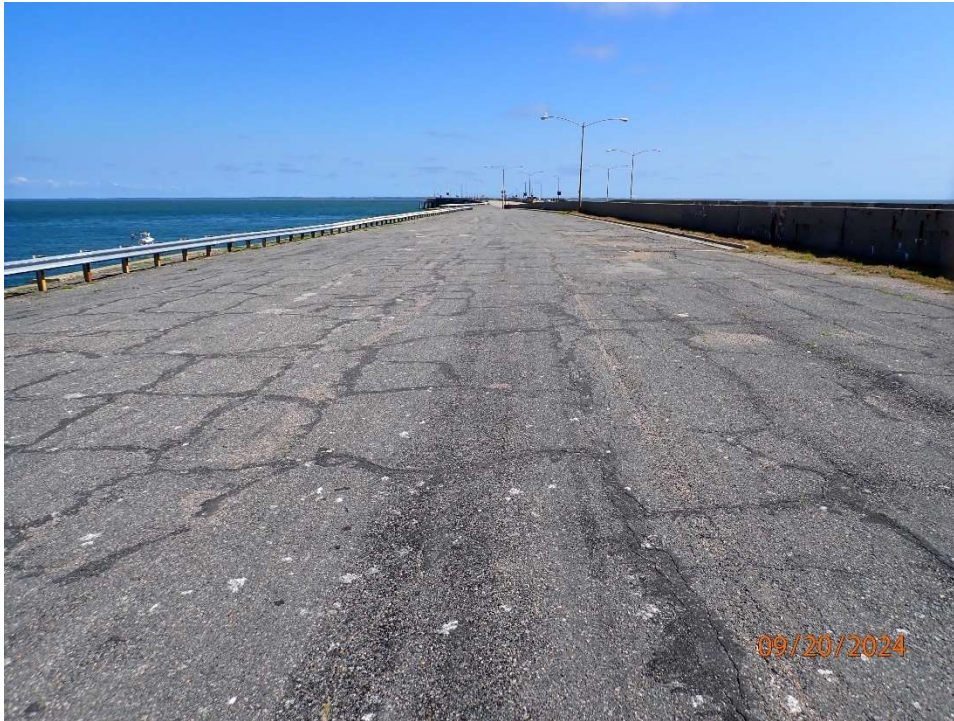
Photo 116: Portal Island 4 Surface; typical asphalt condition on portal island.
