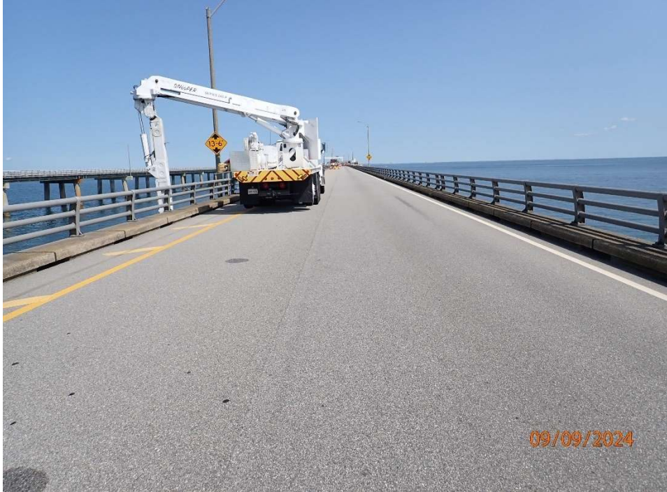
Photo 1: ASB188 Asphalt Wearing Surface – Typical good condition of wearing surface.
