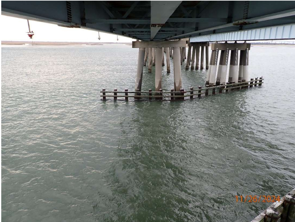
Photo 67: FINB2 Substructure and fender system in small boat channel.
